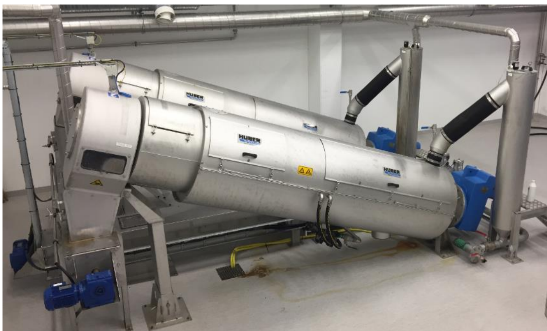
Figur 11: Skruepresser for slamavvanning, Hartevatn RA
